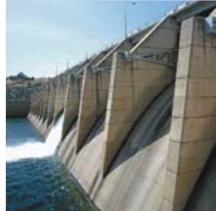
Thermalito Diversion Dam Powerplant
