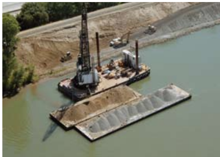
Levee repair site on Sacramento River
