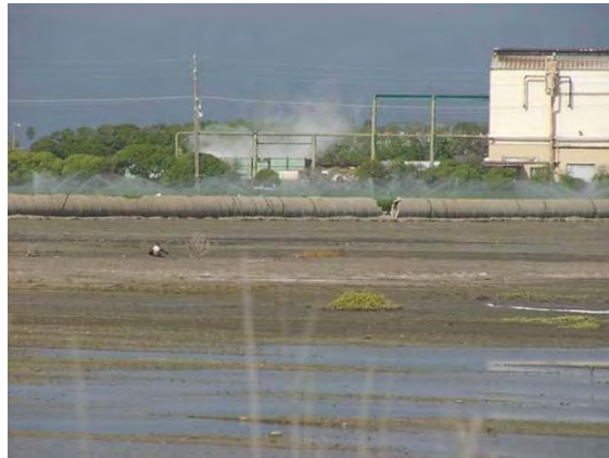
Historical Sewer Pipe in MWD/Oxnard Property Source: David Pritchett
