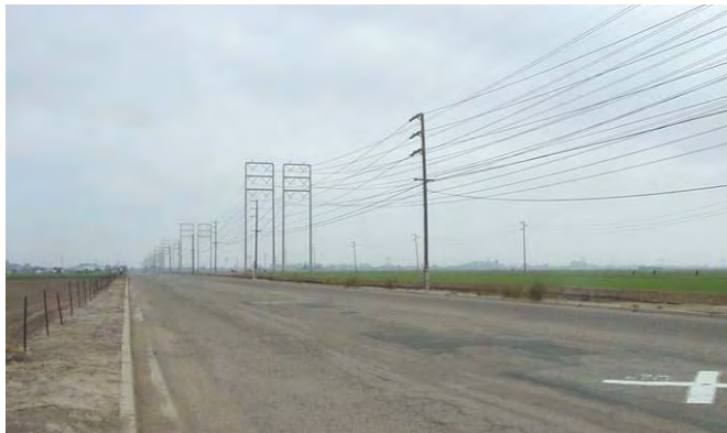
Power lines along Edison Drive (looking north)
