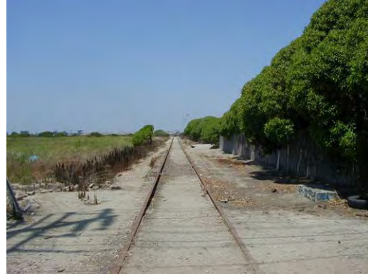
The north-south running spur terminates at the Oxnard Beach Generating Station (viewing north near McWane Boulevard)
